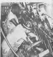
ELECTRICIANS, LEFT, work on the main generator as assistants delve into the intricacies of her main propulsion. A bow fender supports, details of which are shown in the circle, the Esso San Nicolas fills the berth just as prepares for a similar overhaul amidst the scaffolding for return to service this past
